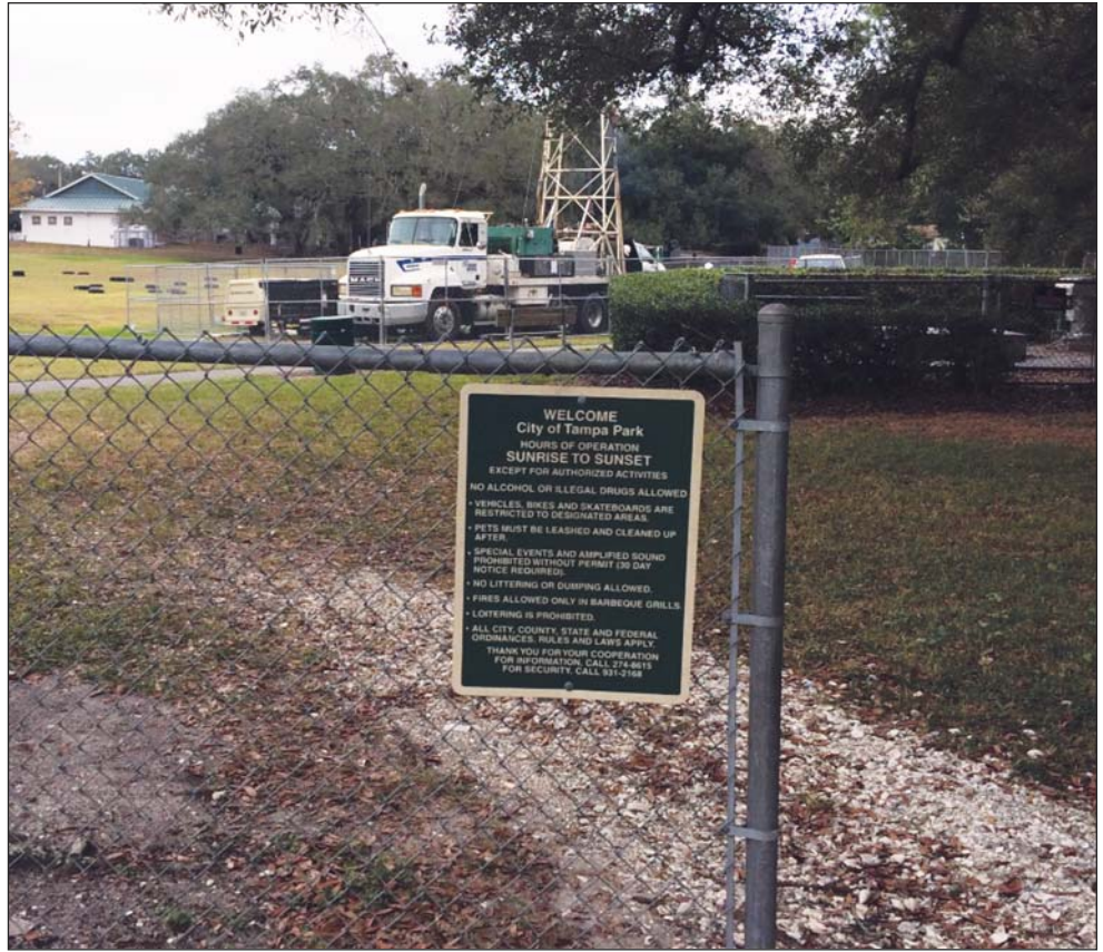
Figure 5. Drilling an Exploratory Core at the Woodlands Terrace Park Site
